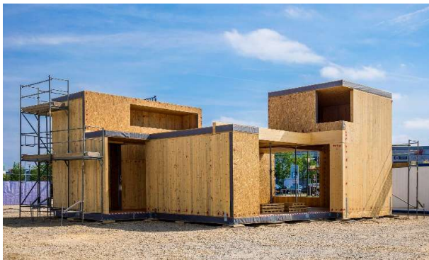
Fig. 2. House EFdeN Signature modular wooden structure
